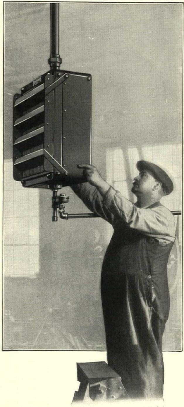
*The illustration shows how simple it is to DIRECT THE HEAT from the Modine Unit Heater WHERE NEEDED — toward a bad door or window, lathe, work benches, etc. One man with a wrench does it in a few minutes' time.*
