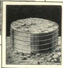
Inside that tapering shell of spirally reinforced steel every Raymond Concrete Pile takes its exact length and taper—and keeps it—because every shell is left in place in the ground. This is THE famous Raymond Method for speed, certainty and safety.
