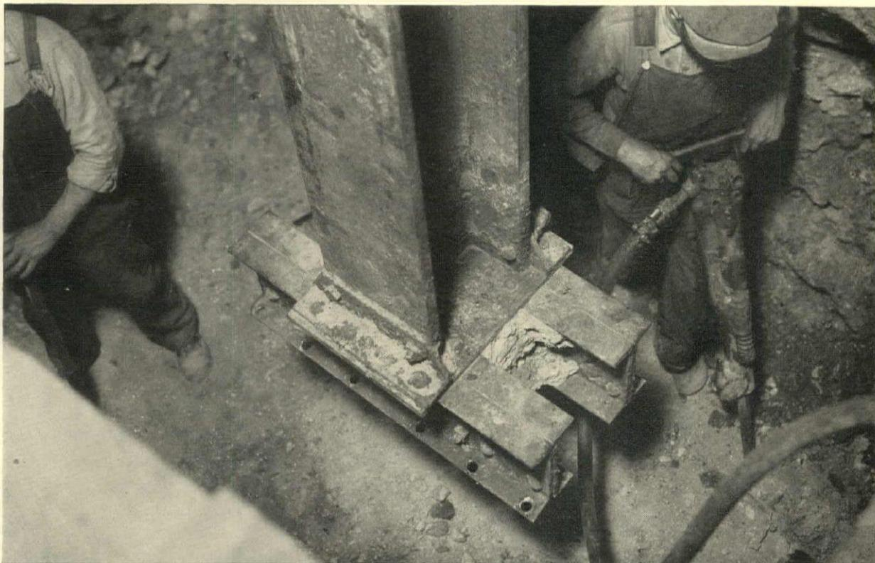
EXCAVATING FOR NEW FOOTING UNDER AN EXISTING COLUMN
