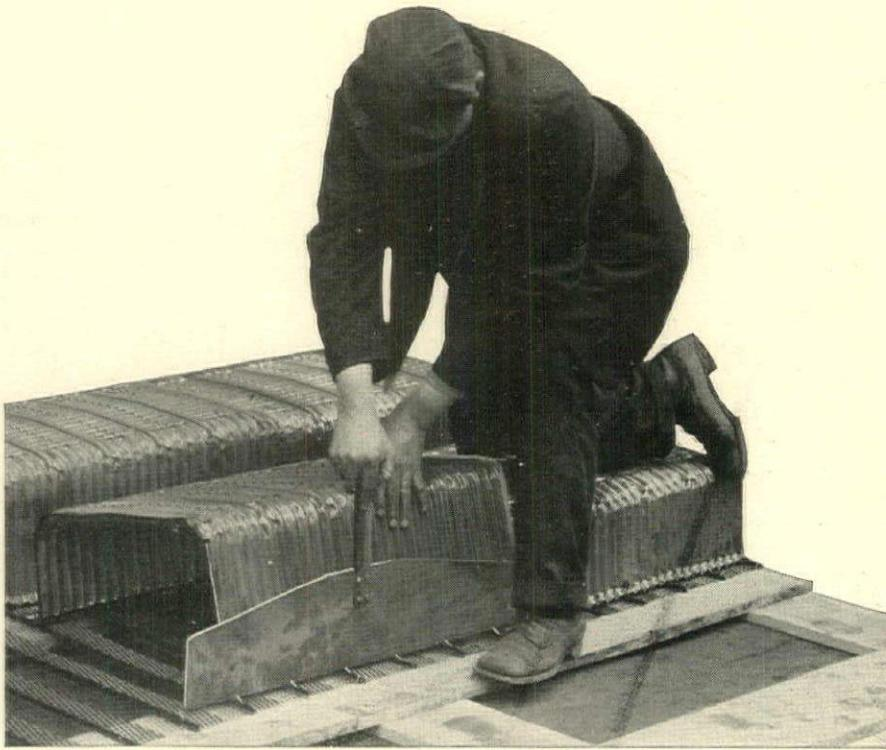
Truscon Floretyles are sprung into prongs in the Locktyle Lath. A fast, labor-saving type of construction.
