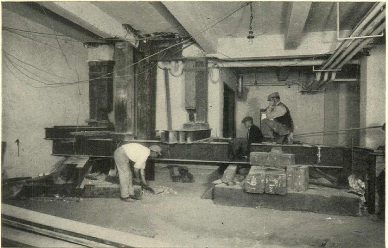
SHORING GIRDERS AND BEAMS IN BASEMENT TO PERMIT EXCAVATING FOR NEW FOOTING UNDER EXISTING COLUMN
