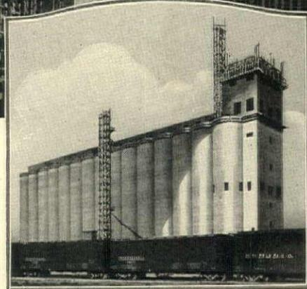
Grain elevators comprise only one of the many types of structures that are advantageously built of that high strength combination, concrete and rail steel reinforcing bars.
