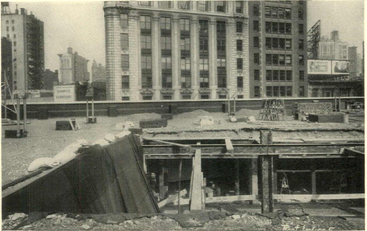
ROOF OF COLONNADE BUILDING SHOWING COURT OPENED FOR CONSTRUCTION. NOTE WATERPROOF BOXES OVER COLUMN STUBS TO PROTECT LOWER STORIES FROM THE WEATHER
