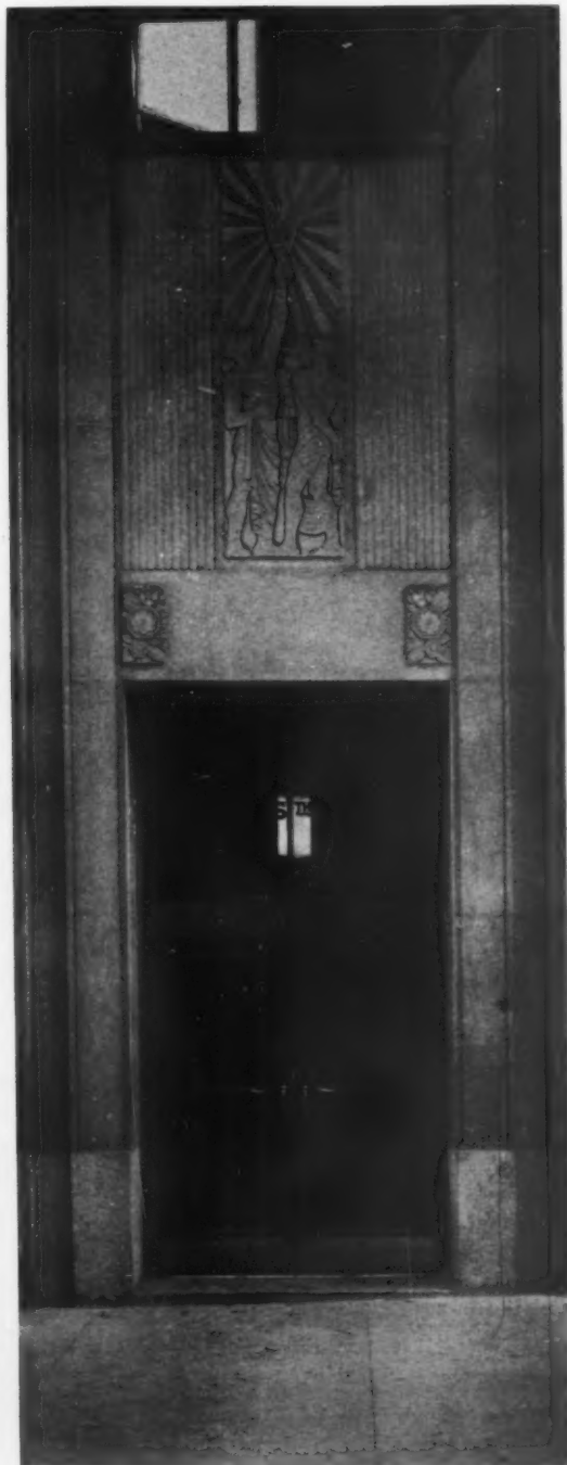
DETAIL OF MAIN ENTRANCE TO BUILDING
