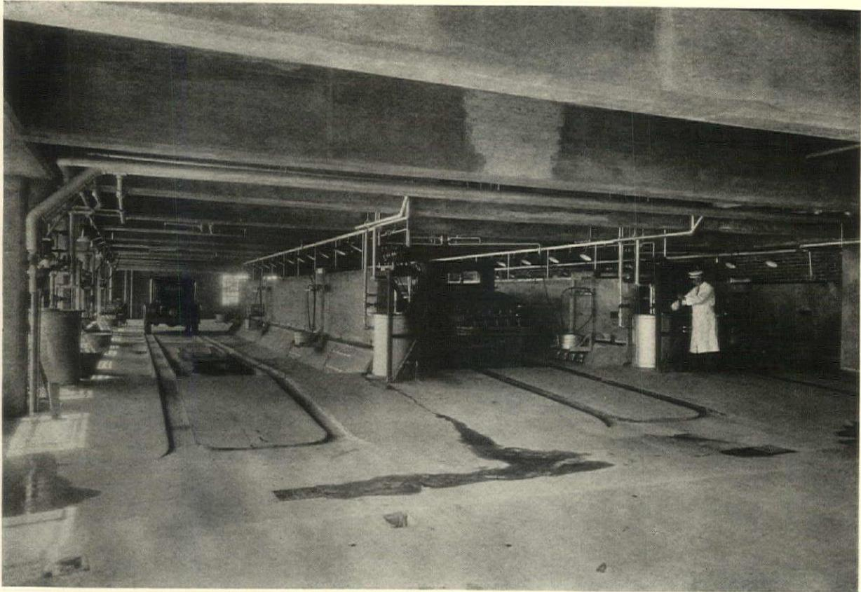
WASH RACKS, SHOWING MOVABLE WASHING EQUIPMENT ON OVERHEAD TRACK
