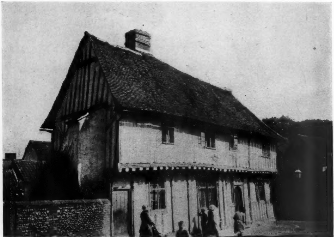
OLD HOUSE AT LAVENHAM, SUFFOLK
