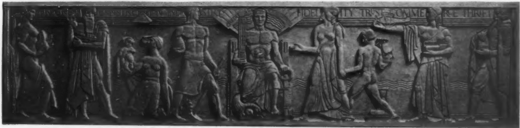
PANEL EXECUTED IN LIMESTONE, 6 FEET BY 25 FEET, LOCATED THIRTY FEET ABOVE SIDEWALK
