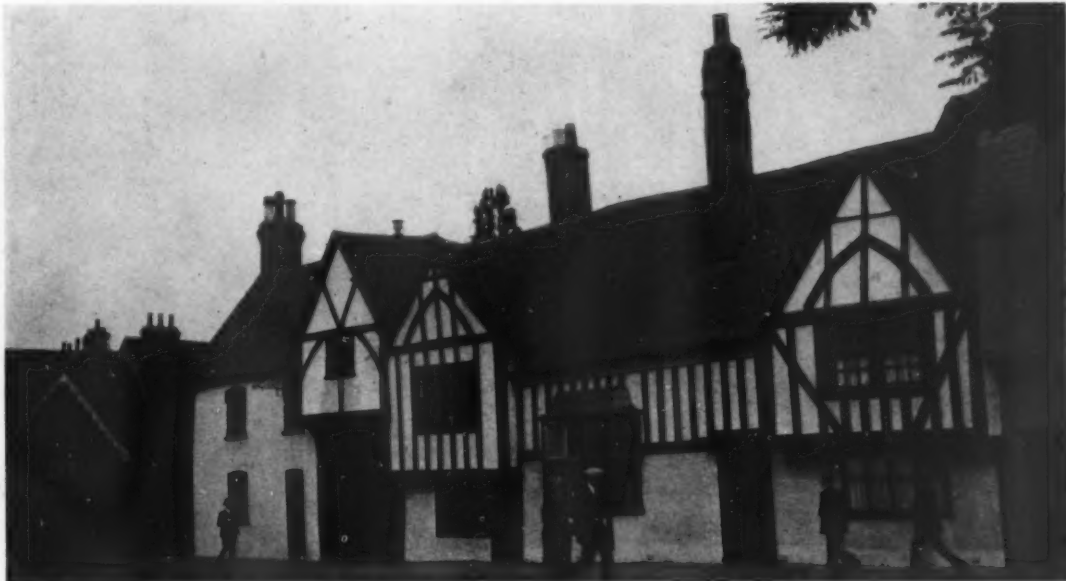
IN THIS EXAMPLE OF BAD RESTORATION AT HITCHIN, HERTS, THE OLD TIMBERS AND BAY ARE PAINTED SHINY BLACK AND THE STUCCO AND BRICKWORK PAINTED WHITE
