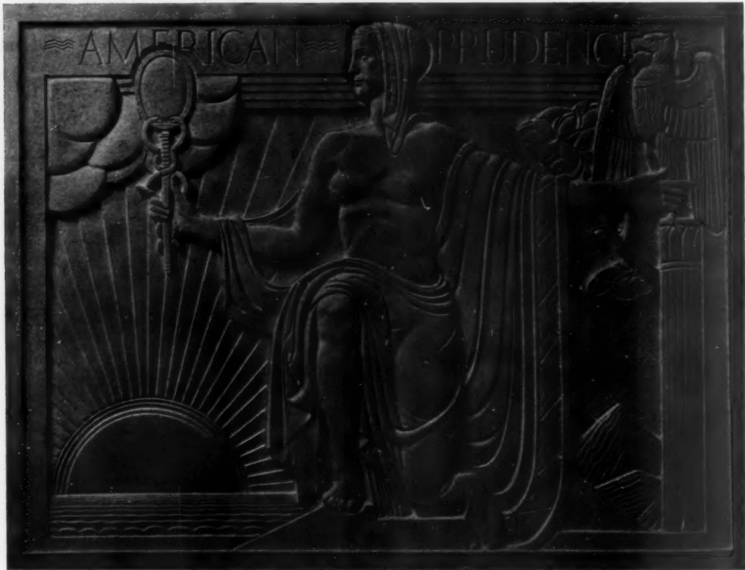
PANEL ABOVE SIDE ENTRANCE EXECUTED IN LIMESTONE. SIZE ABOUT SIX FEET BY EIGHT FEET SCULPTURE DESIGNED AND EXECUTED BY LEO FRIEDLANDER. DAVIS, DUNLAP AND BARNEY, ARCHITECTS
