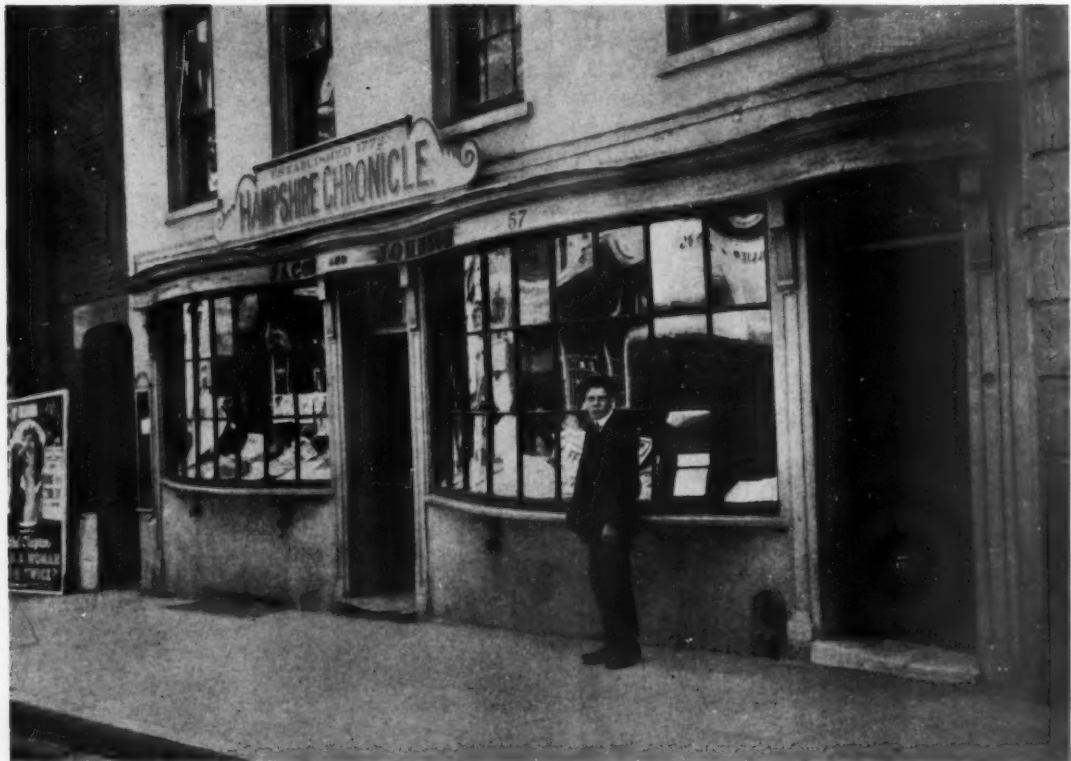
SHOW WINDOWS MADE UP OF SMALL PANES ARE INTRIGUING, EVEN THOUGH VISIBILITY IS SOMEWHAT IMPAIRED IN COMPARISON WITH THE MODERN PLATE GLASS SHOP WINDOW
