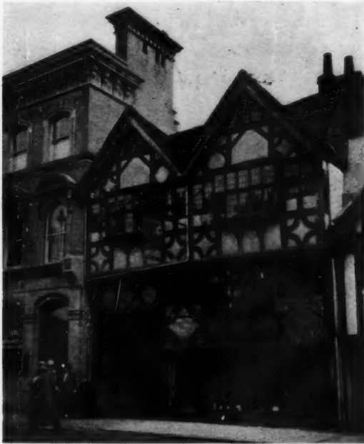
OLD SHOP AT FARNHAM, SURREY NOTE THE MODERN ATROCITY NEXT DOOR
