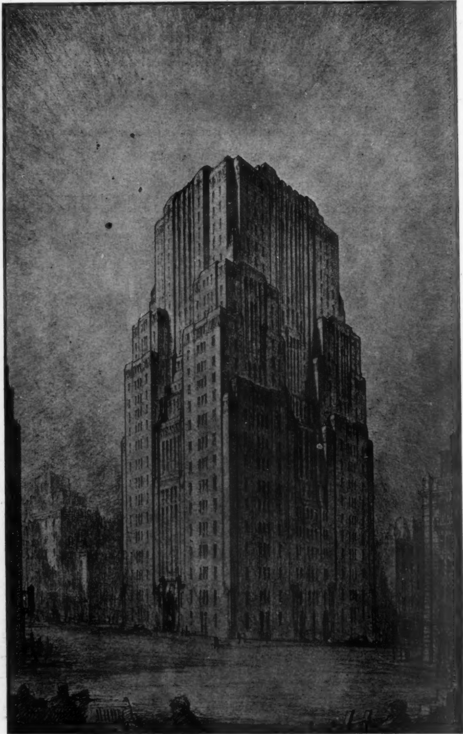
SOUTHERN BELL TELEPHONE & TELEGRAPH COMPANY BUILDING, ATLANTA, GA.
