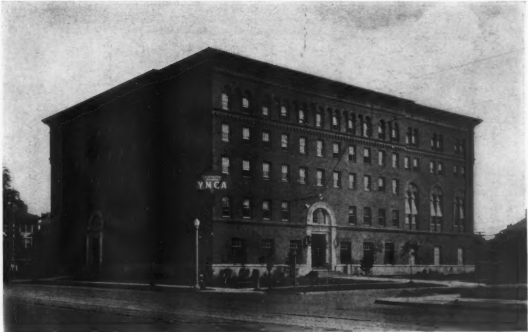
GENERAL VIEW OF EXTERIOR
