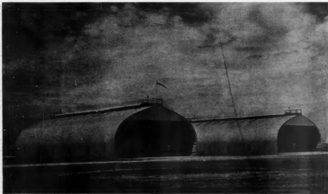
STEEL HANGARS, HOUSTON AIRPORT, HOUSTON, TEXAS
