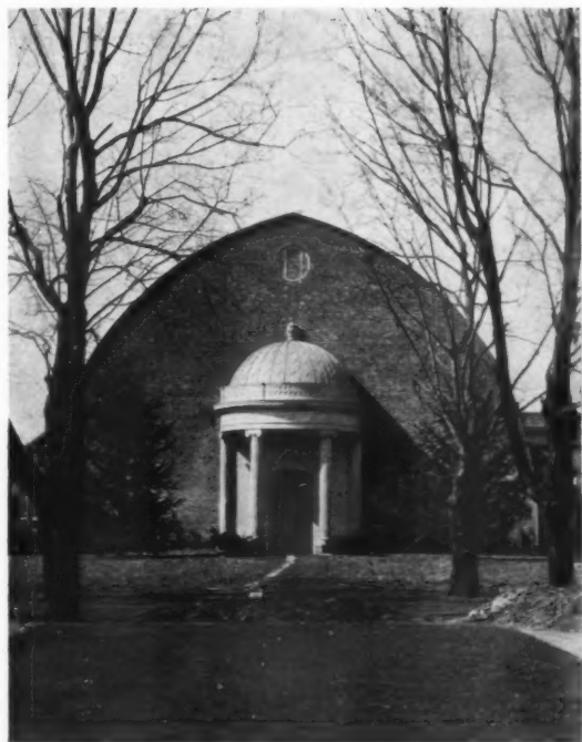
HARRISON WILLIAMS' ENCLOSED TENNIS COURT BAYVILLE, N. Y.—DELANO & ALDRICH, ARCHITECTS
