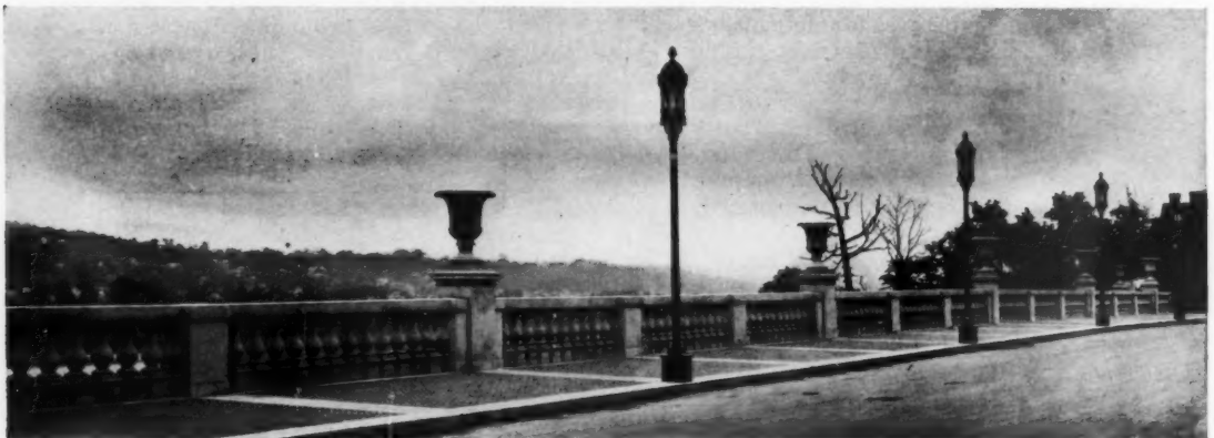
BALUSTRADE AND LIGHT POSTS, HETHS RUN BRIDGE, HIGHLAND PARK, PA.
