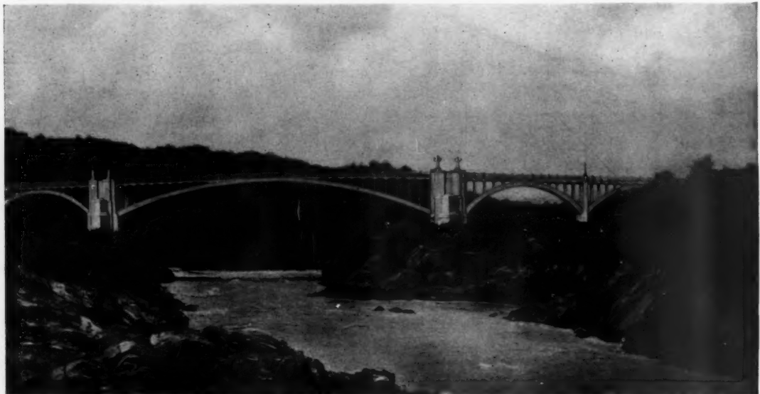
PROPOSED BRIDGE ON THE POTOMAC RIVER, AT GREAT FALLS, WASHINGTON, D. C. MEIGS, LONG & BEALE, ENGINEERS
