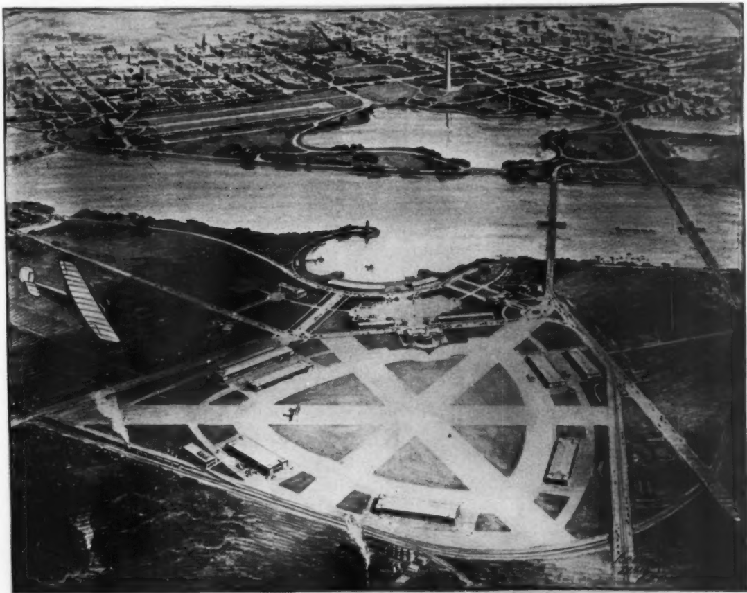
AIRPLANE VIEW OF THE PROPOSED DEVELOPMENT OF WASHINGTON AIRPORT FROM THE ORIGINAL DRAWING BY SCHELL LEWIS
