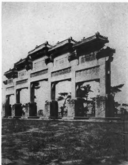
MARBLE PAI-LO, OR MONUMENTAL GATEWAY, MARKING ENTRANCE TO EASTERN TOMBS. TYPICAL OF THIS WIDELY USED ELEMENT. LESS IMPORTANT ONES AT THE ENTRANCES OF PRIVATE CEMETERIES AND AT INTERSECTIONS OF PROMINENT STREETS ARE OF WOOD. THIS IS AN INTERESTING EXAMPLE OF THE EXECUTION IN STONE OF STRUCTURAL MOTIFS DERIVED FROM WOODEN PROTOTYPES.
