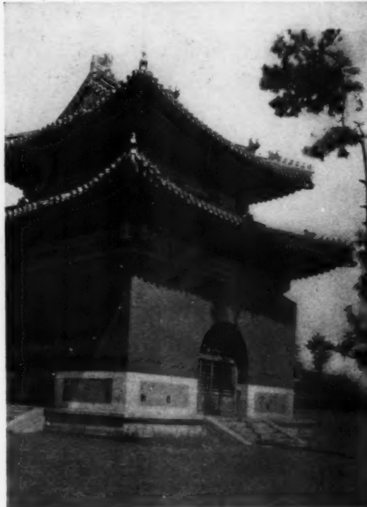
ONE OF TWO TABLET-HALLS MARKING APPROACH TO A TOMB. THE MASSIVE CORNER PIERS LEAVE THE INTERIOR A GREEK CROSS IN PLAN. WITHIN IS AN ENORMOUS TORTOISE OF WHITE MARBLE, THE TORTOISE BEING A SYMBOL OF LONGEVITY OR ETERNITY. FROM HIS BACK RISES A LARGE RECTANGULAR STELE ON WHICH CAREFULLY INCISED MANCHU AND CHINESE WORD-CHARACTERS IN APPROPRIATE PROFUSION TELL OF THE VIRTUES AND OF THE REIGN OF THE IMPERIAL INCUMBENT.
