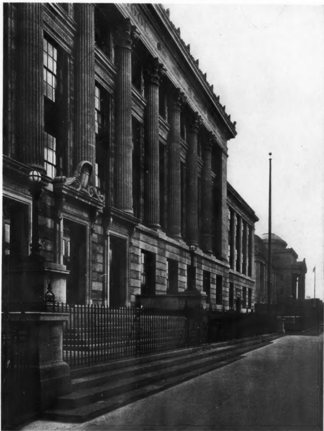
CATHOLIC HIGH SCHOOL, BROOKLYN, N. Y. ROBERT J. REILEY, ARCHITECT
