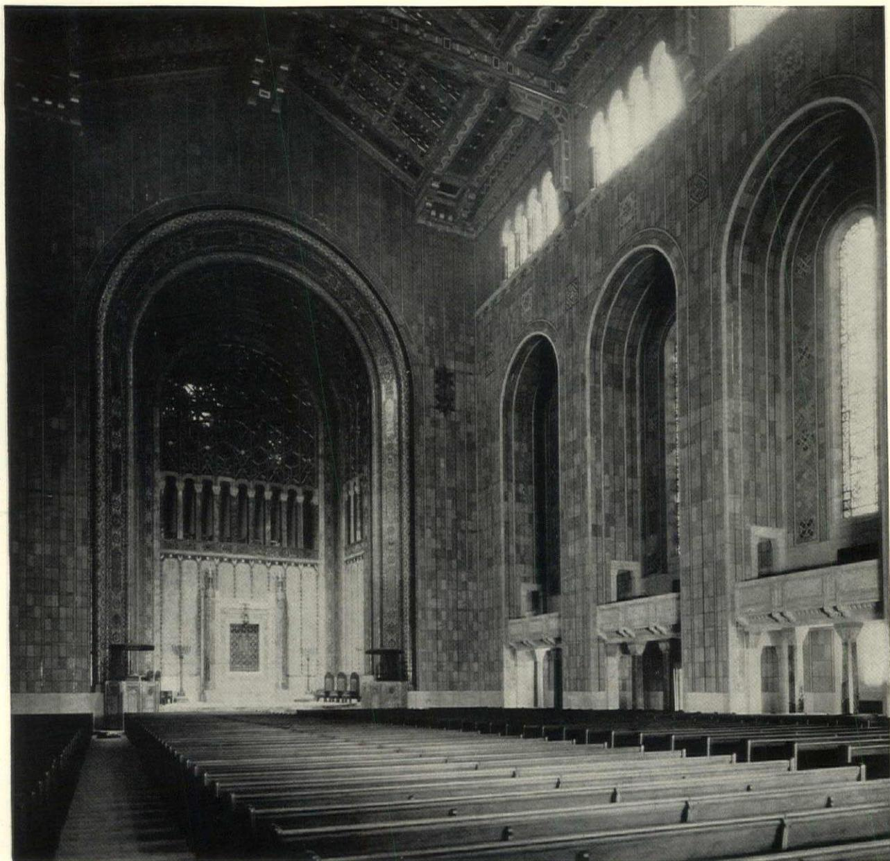
A SIDEWALL INSTALLATION OF AKOUSTOLITH SOUND-ABSORBING STONE IN TEMPLE EMANU-EL, NEW YORK CITY, IN A GRADATION OF COLOR FROM LIGHT AT THE BASE TO DARK AT THE CEILING AND WITH GOLD CERAMIC INSERTS.
