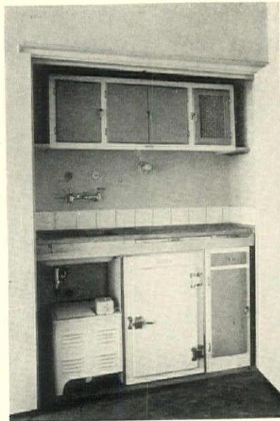
*Service pantries have a refrigerator designed by the architects and are provided with an unusual amount of working space for a unit of this type*
