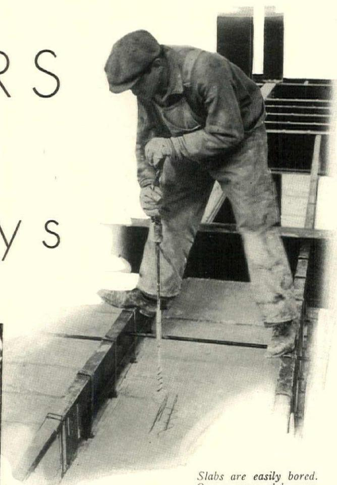
*Slabs are easily bored. One or more slabs may be omitted as desired and laid later when circumstances require*
