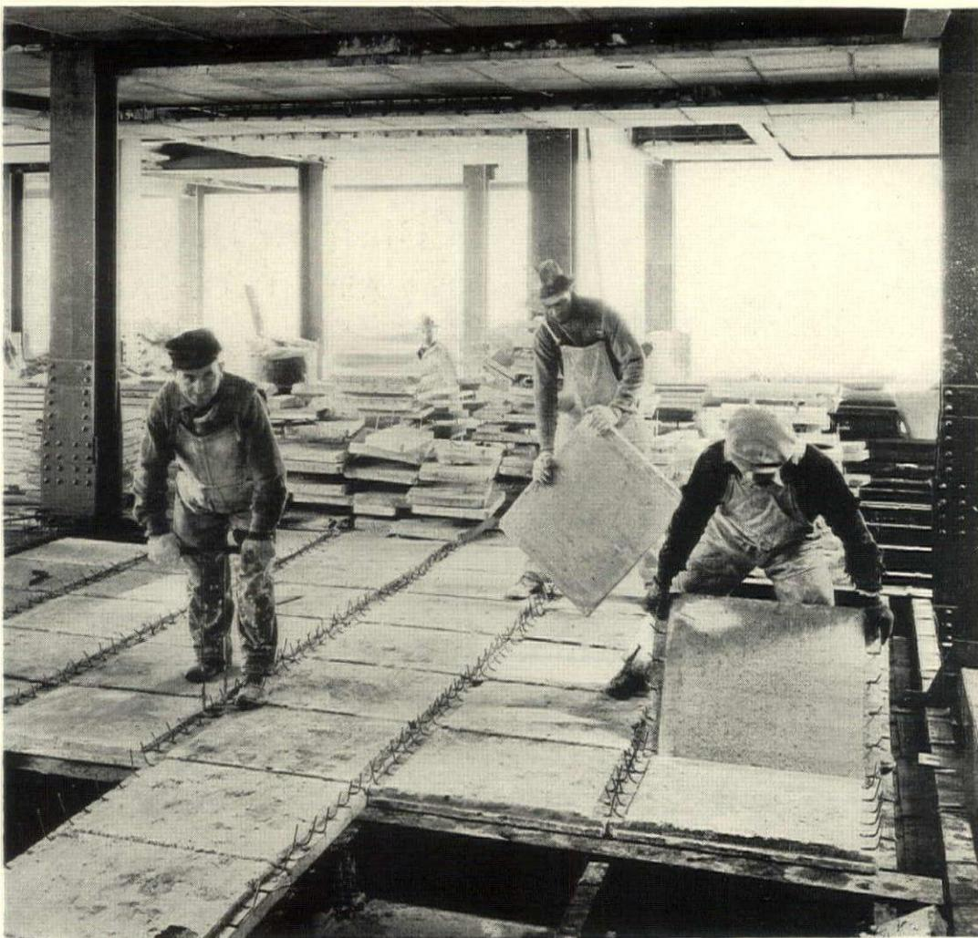
flange and is tightly clamped to it by steel straps. The haunches are then formed with 2" solid gypsum blocks.
