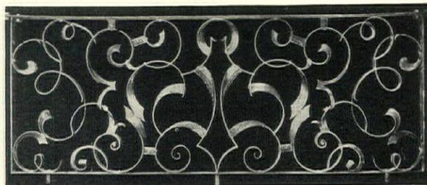
*Two sections of the rail in the main stairhall of the Justice Building in Hamm in Westphalen, Germany, designed and executed by Carl Wyland of Cologne. Herr Warnemunde of Hamm was the architect. From "Moderne Bauformen" issue of May, 1930*
