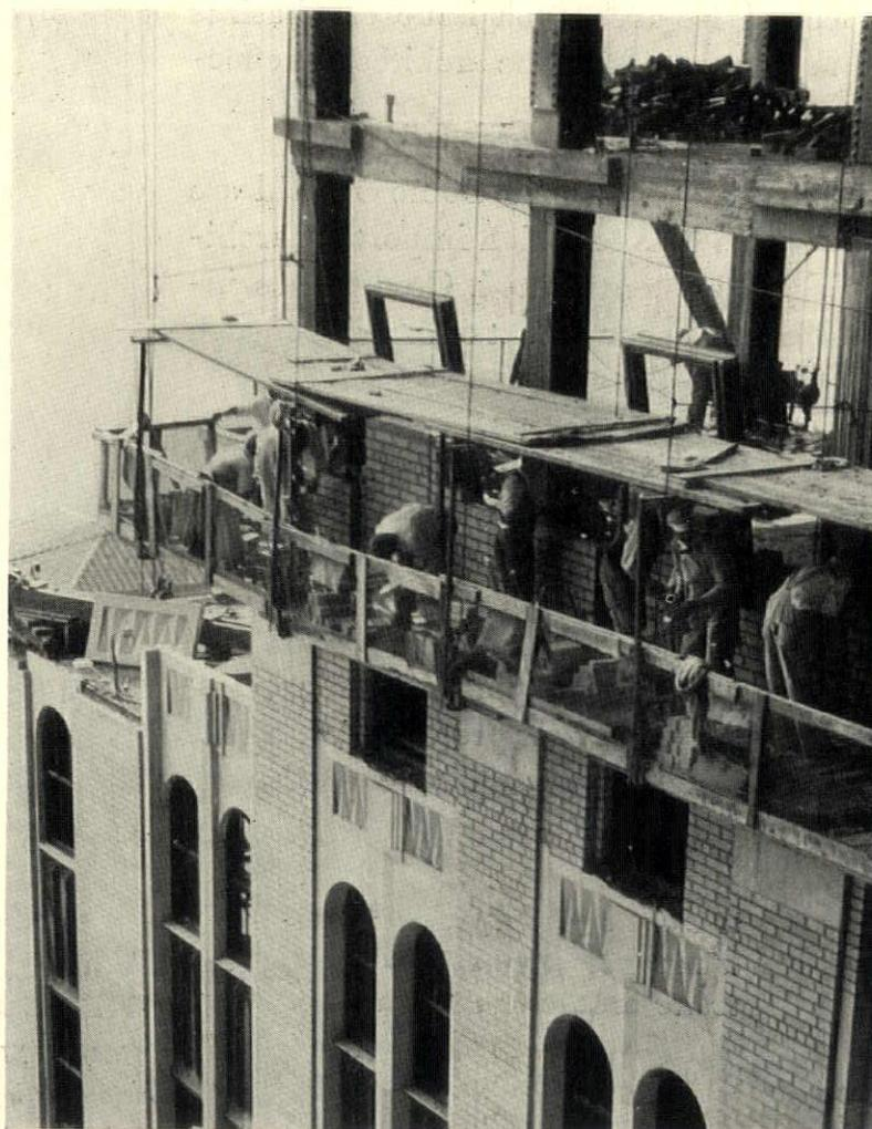
Laying up Waldorf Grays on an upper story of the Waldorf Astoria. Note size of units compared to standard bricks. Mortar is still fresh in this photograph—dries out to same color as brick.
