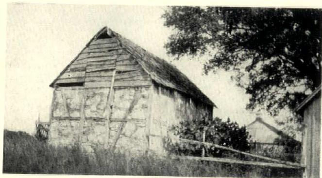
Half timber and stone nogging with wide joints of white mortar
