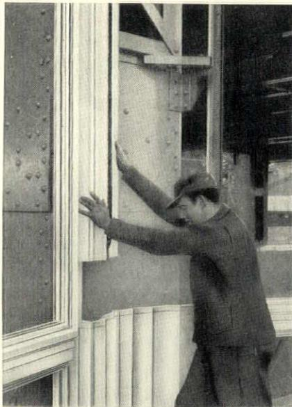
Extruded aluminum window and pier construction and erection method—also the expansion joint provided at each floor.
