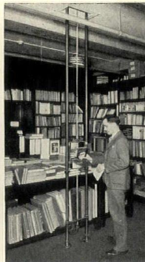
Main floor view of Sedgwick Lift used for handling books between main floor and the mezzanine. Various styles of carrier available to meet specific needs.
