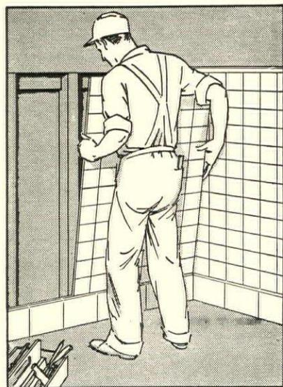
Waltiles' 32" x 48" x 3-16" sheets can be cut to fit any wall surface. Standard sheets are scored every four inches and are also furnished in 8" x 8" and 16" x 16" scoring. In new houses it may be invisibly nailed directly to the sheathed studding, saving lath and plaster. Waltile plastic compound is furnished for application to old plaster walls. Cap and base moulding to match or contrast with sheets are also supplied.
