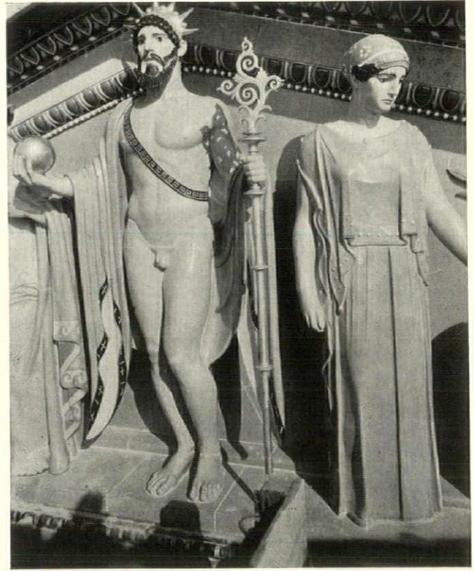
Jointing was successfully arranged to avoid marring the figures. At the left the twelve-foot figure of Zeus has been partly assembled. At the right the joints have been pointed with mortar colored to match the glaze
