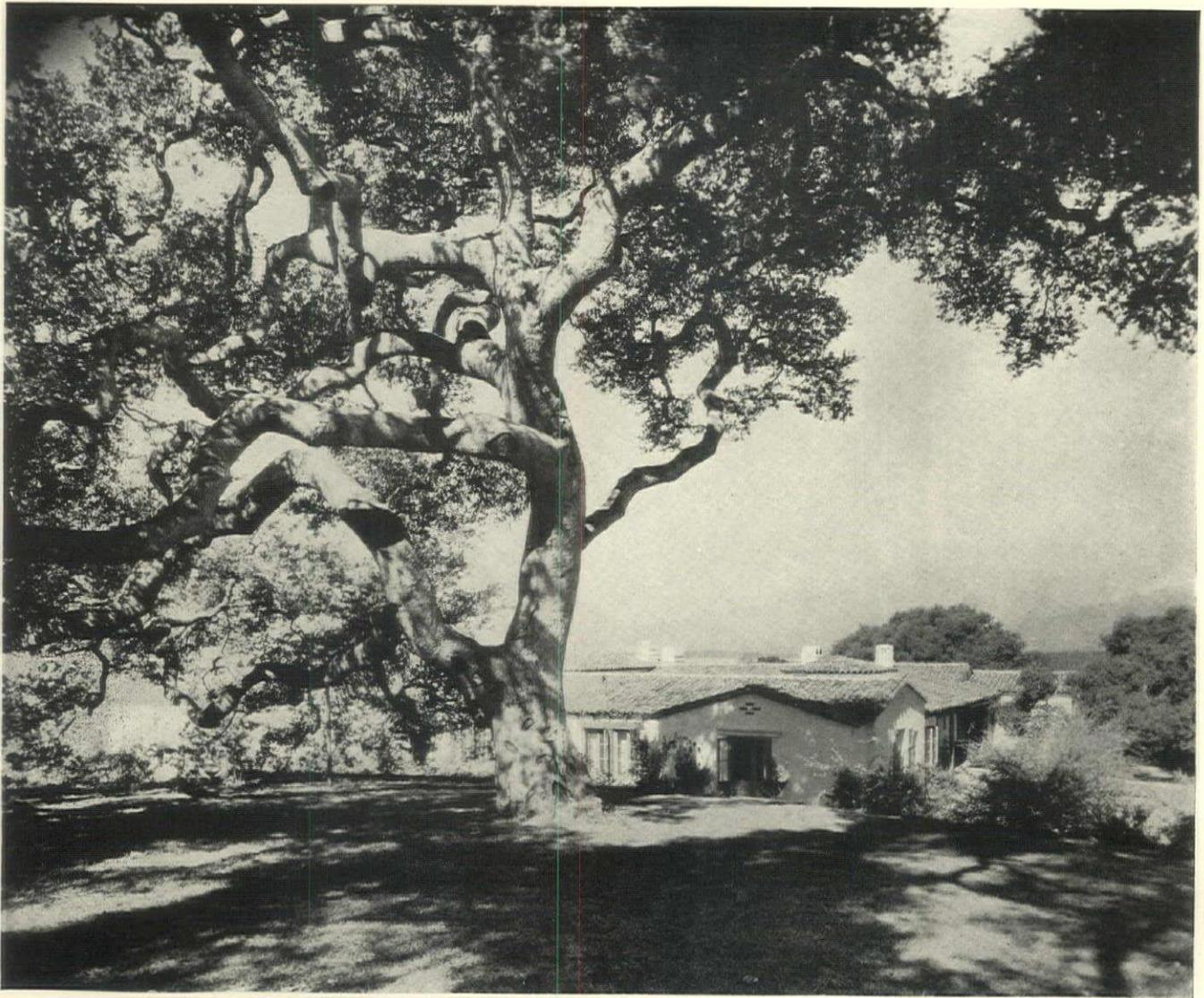
CONSTRUCTION DATA: Wood framing faced with smooth white plaster and some brick veneer painted white. Roof, mission tile, antique finish. Exterior beams, posts, lintels and cornice stained brown. Sash, doors and exterior blinds painted olive green. Outdoor paving and floor of loggia (see page 80), flagstone. Hall floor, red tile. Floors of main rooms are of broad oak boards; other floors are oak of usual width. Living room (see page 80) has plaster walls and an open trussed wood ceiling
