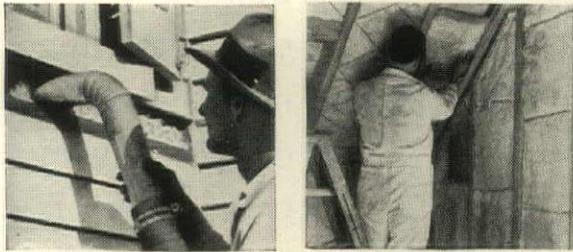
● Left: "Blowing" clapboard house with J-M Type A Rock Wool. Right: Fitting J-M Type B Rock Wool "bats." Either method fills wall spaces completely; leaves no room for circulation of air.
