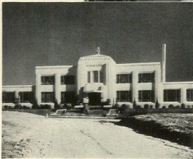
*All exterior ornament cast in place. Surface forms were of plywood with construction joints at designated intervals. Color scheme is mainly a white cement and lime dash coat with ochre color base at the grade line. Entrance steps a bright red.*
