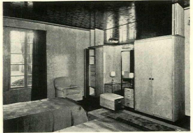
Bed room of a prefabricated house built by the Weyerhaeuser Timber Co. of Tacoma, Washington, that is expected to "revolutionize small house construction." It was built in twenty-one days from structural panels made entirely in the factory. Interior walls and partitions are of plywood in natural finishes. Ceilings are decorated. The house is completely air-conditioned.
