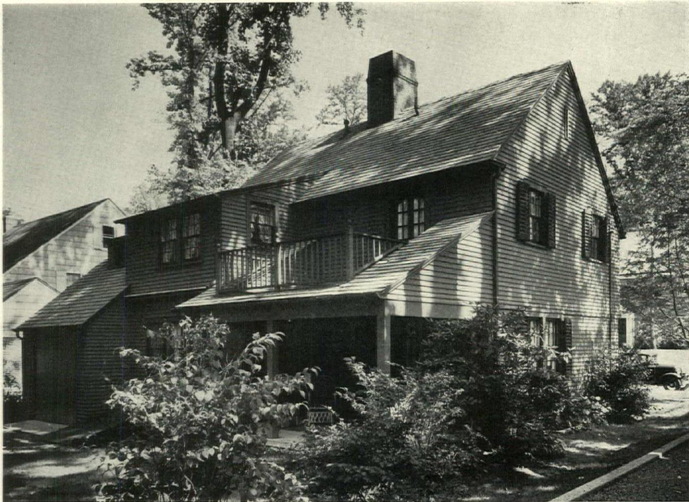
Exterior: Narrow clapboards painted brownish-red. Common brick chimney, unpainted. Dark green shutters. Interior: Rough plaster walls, oak floors. Living room, right, paneled with pine slightly antiqued and coated with dull varnish. House contains 32,000 cubic feet. Cost, in 1932, \$11,000
