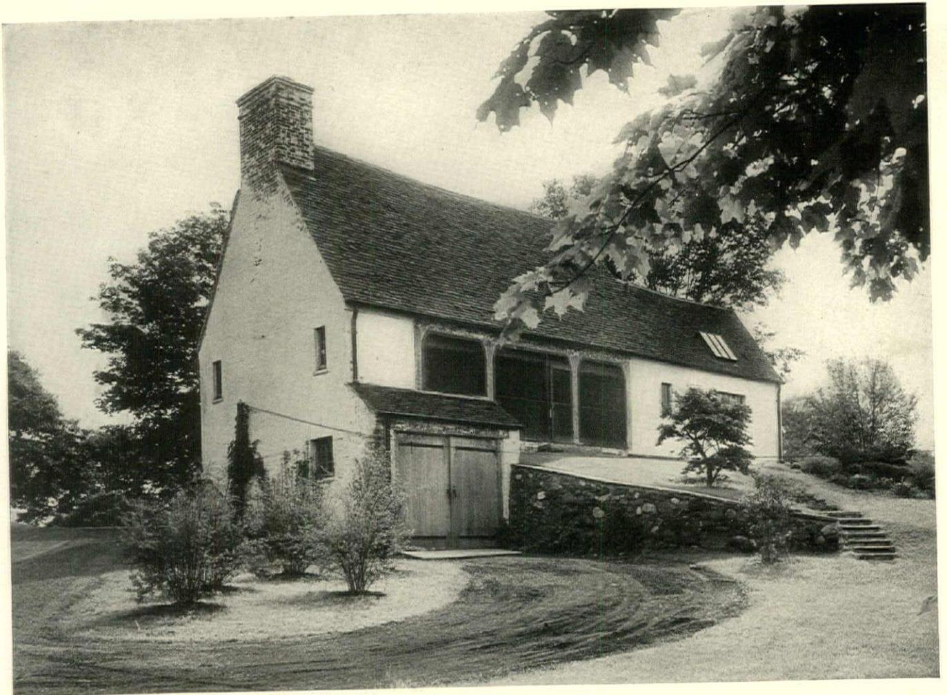
Construction: frame, veneered with white-washed common brick. Roof: red and brown hand-made shingle tiles. Exterior woodwork: solid oak, stained with creosote and white-washed. Interior woodwork: oak and pine, stained brown. Upper floor is used exclusively for recreation, independently of shower and locker conveniences in basement. Consequently no stair between the two floors was necessary.
