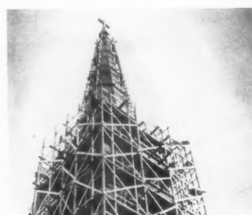
Cathedral of Assumption, Louisville, Ky. Architect: D. X. Murphy and Bros.
