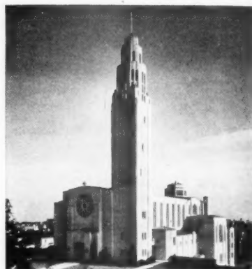
St. Joseph's Church, Seattle. Architects: A. H. Albertson, J. P. W. Wilson, Paul Richardson.
