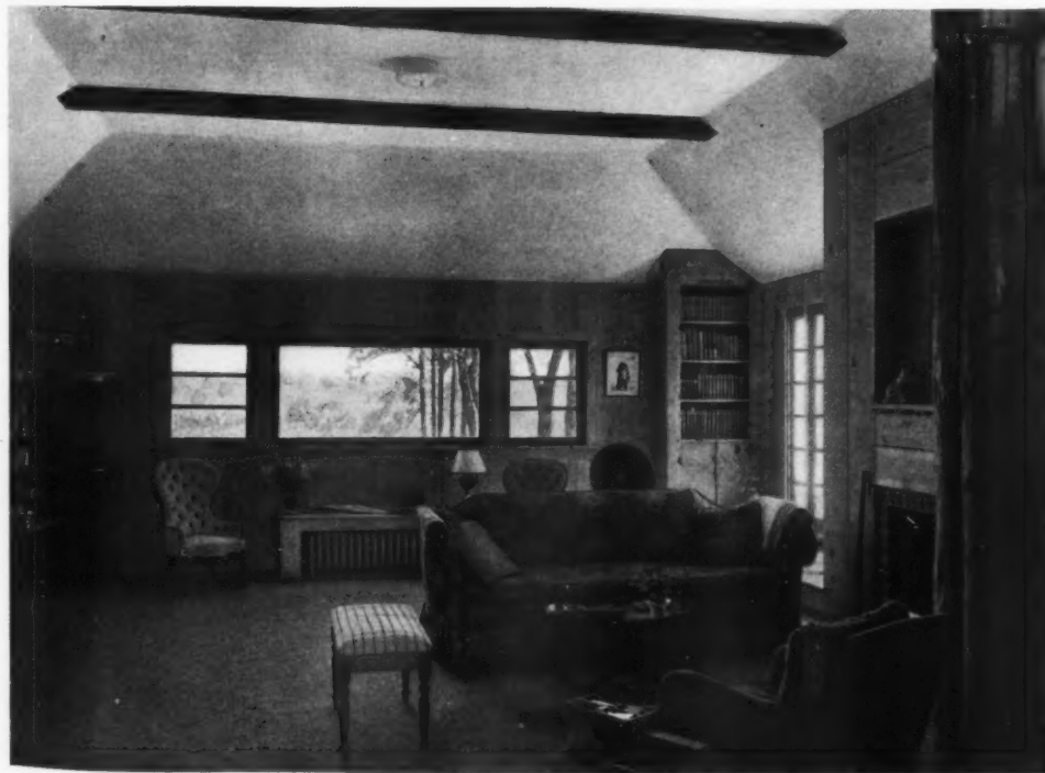
HOUSE OF DENNY BRERETON GREENWICH, CONN. ALLAN TAFT SQUIRE, ARCHITECT
