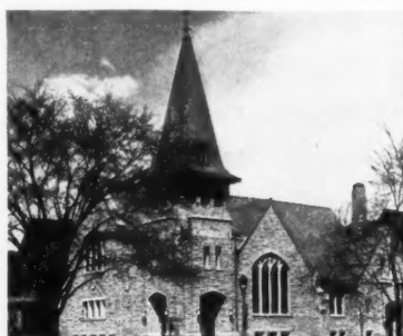
St. Paul's Lutheran Church, Milwaukee. Architect: Hugo Logemann.
