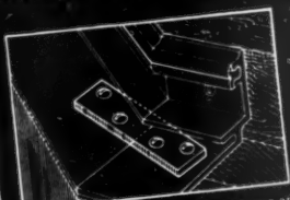
Heavy metal cleats seated in groove at corners secure miter against rising, falling or spreading due to faulty frame work.
