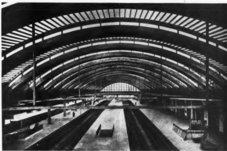
Above: model of exhibition house to be built in Miami Beach, Fla. Robert Law Weed, architect. Above, right: a huge turntable upon which cars revolve about a center service station is a new time and space-saving device. Right: concrete rib troughs facilitate cleaning of roof windows in the new train shed at Reims, France
