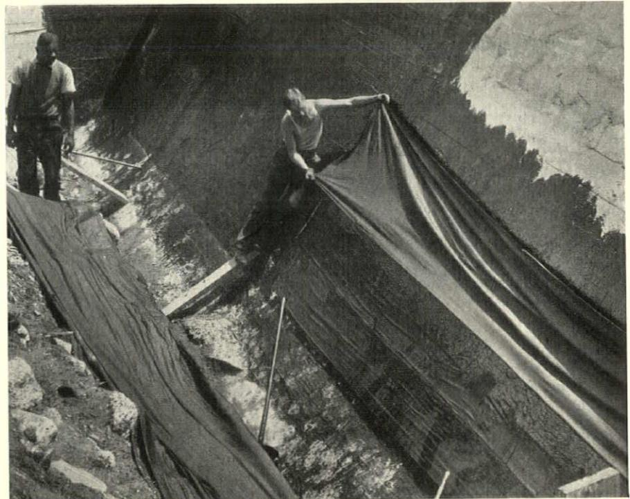
**Figure 2 . . .** Membrane waterproofing consisting of plies of fabrics or felts embedded in hot moppings of pitch or asphalt are used wherever vibration, settlement or cracking of masonry may occur
