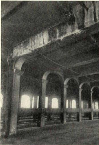
Concrete spalling on a two-level bridge in an eastern city. The waterproofing disintegrated.\*
