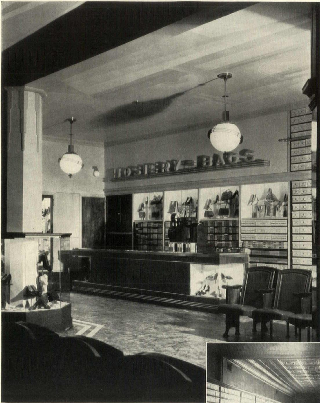
Modernization of this shoe store is typical of possibilities in nearly every city in the country. On the exterior (facing page) an obstructing column was removed from the entrance, show windows were enlarged, the facade faced with Vitrolite and trimmed with aluminum. On the interior the new floor is linoleum; walls and ceilings painted cement plaster; lighting fixtures chromium trimmed with black. Cases and furniture are walnut with chromium trim
