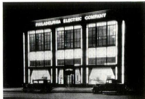
Built-in luminous elements which provide desired lighting effects at night, may readily be made an integral part of the daytime composition. Here flashed opal and ground glass spandrels and bandings overlaid with bronze grilles become important decorative features. John T. Windrim, architect
