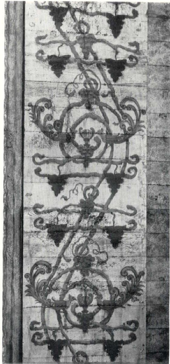
**COLOR STAINS**, unlike oil paint applied to concrete, penetrate the pores of the material, thus becoming, in fact, a homogeneous part of the structure. As in the interior decoration of St. Joseph's Church, Seattle, the use of stain colors permits simplicity of structure and richness of surface treatment without sacrifice of the monolithic characteristics of the design. A. H. Albertson, architect; Joseph W. Wilson and Paul Richardson, associate
