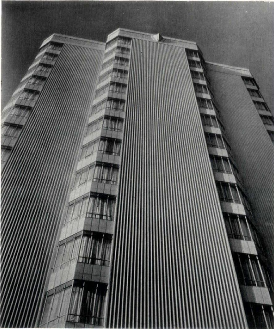
**TEXTURE** through form and scale obtained by using black corrugated iron as a form liner. Only two form sections were used, the lower one being removed when the concrete had hardened and replaced in perfect alignment above the upper one. Complete lack of joint lines visibly demonstrates the monolithic character of the construction. Edmond Meany Hotel, Seattle, Washington. R. C. Reamer, architect
