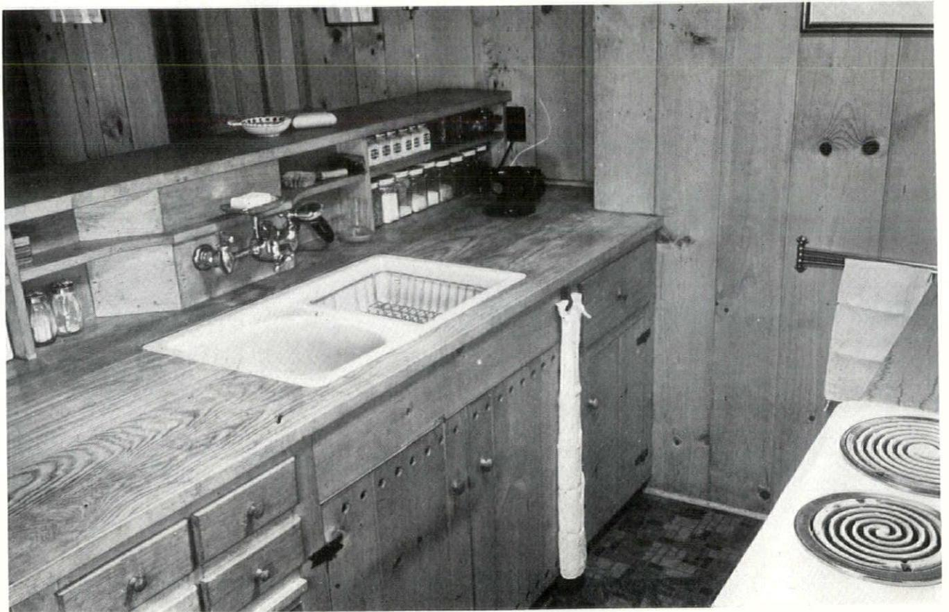
In the Hoyt Catlin kitchen are 32 square feet of working top, within two steps of the center of the room. Working surfaces are 36 inches high from floor and 22 inches deep, front and back
