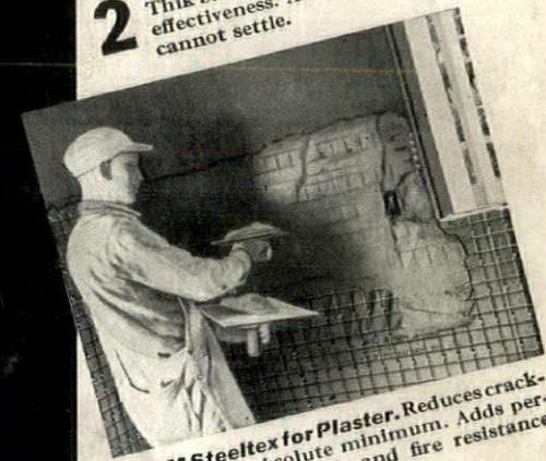
**3 J-M Steeltex for Plaster.** Reduces cracking to an absolute minimum. Adds permanence, strength and fire resistance.
