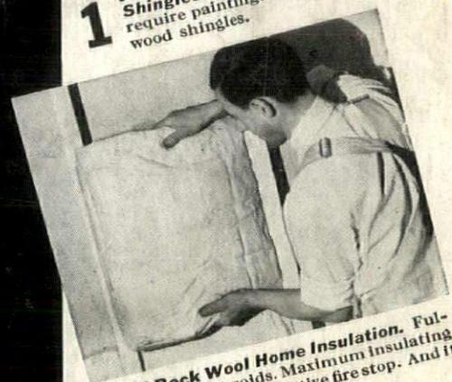
**2 J-M Rock Wool Home Insulation.** Full-thick bats. No voids. Maximum insulating effectiveness. An effective fire stop. And it cannot settle.
