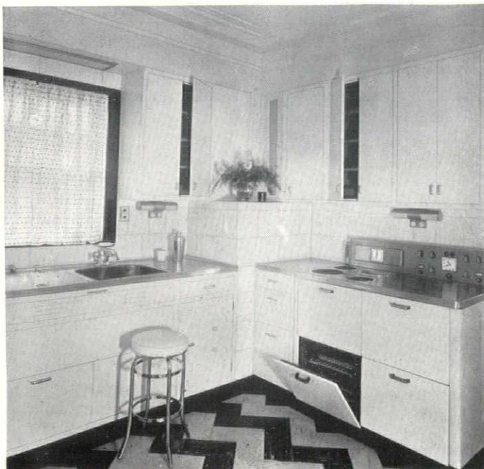
Remodeled kitchen by Louis Andre Lamoreux, Architect, Mansfield, Ohio. Walls, Carrara glass; floor, rubber tile; cabinets, enameled steel. Note soffit lighting over sink and combination convenience outlets and under cabinet lights
