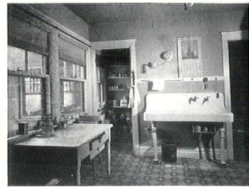
Elimination of storage closet door permitted continuous work top from sink to range. Note linoleum floor turned up into toe-space under cabinets, and ventilation through furred ceiling beam
