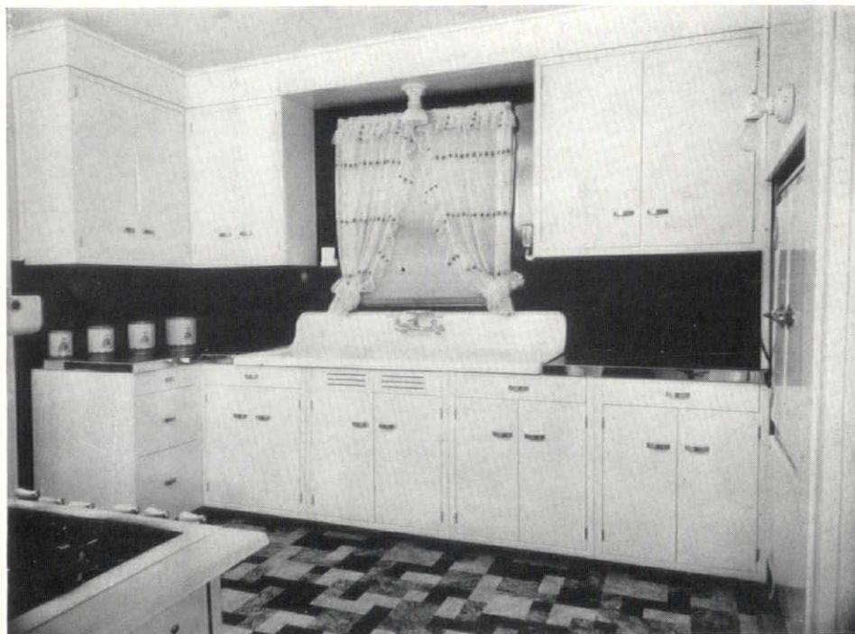
Shifting the sink and adding metal cabinets for adequate storage organized this kitchen. Floor, linoleum; work surfaces, metal; sink, porcelain iron
