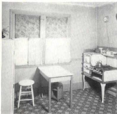
Range and refrigerator have changed places to simplify routine in this kitchen. Note cove base under sink unit, and metal corners protecting synthetic tile wainscot
