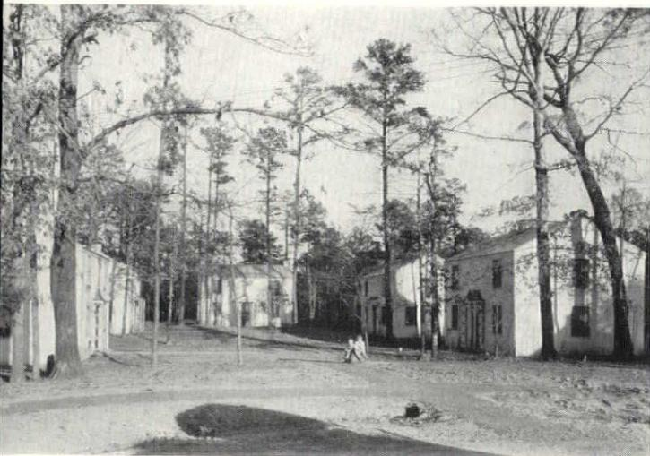
These houses (Types C and D) are built of cinder block with no other finish than paint, both inside and out. Floors are precast concrete slabs on reinforced concrete joists. Heated by coal stoves
