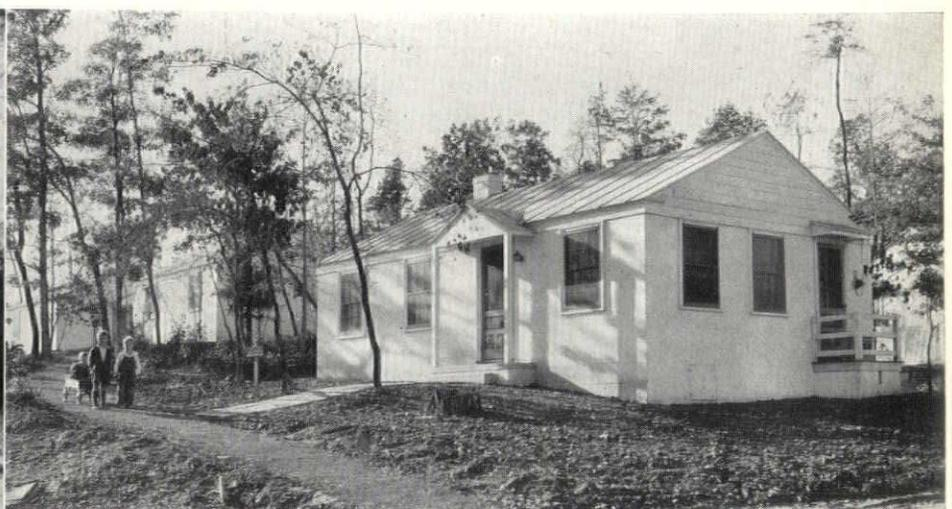
Four-room houses of cinder block (Type A) with paint finish. Floors are concrete slabs and roofs of metal. They are vermin and termite proof and also fire-resisting. Thirty such houses, with numerous exterior variations, were built
