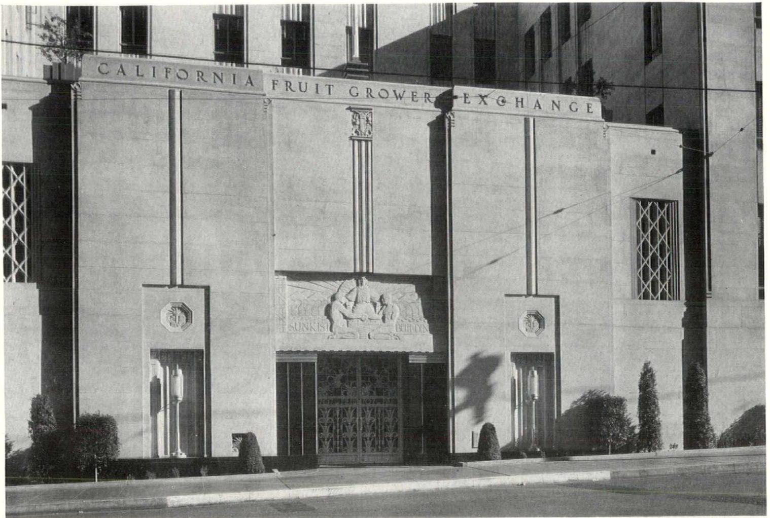
The garage surrounds the main foyer on the ground floor. The large board room without windows on the second story results in a unity of mass at the main entrance. Concrete forms were constructed of plywood in panel sizes. They were rigidly braced to assure exactness of surface in both directions. After stripping the surfaces were stoned and washed down to a uniform color and texture. Spandrels were acid stained
