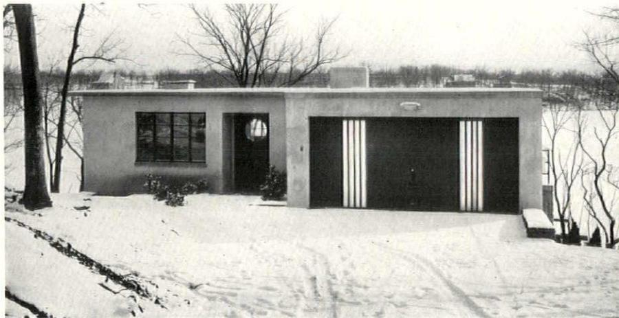
Native stone is used for the first story and foundation walls, while stucco finished concrete block is used for the second story walls. Floors and roof are of concrete slab. Windows are steel casement. All interior walls have plaster finish except in playroom where stone is pointed with white cement joints
