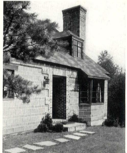
8" and 4" cinder-concrete blocks, unpainted, form an interesting horizontal pattern. Joists are 8" pre-cast concrete. Cost \$7,200
