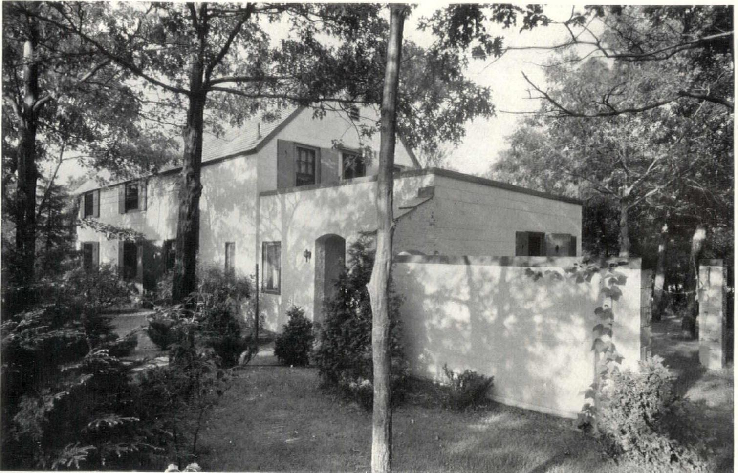
This house of painted concrete block was built in three stages. The terrace over the kitchen is a reinforced concrete panel waterproofed with asphalt and finished with slate
