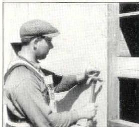
*Celotex sheathing spans four studs—meets on the stud—provides a stronger, better-braced, more wind-tight wall.*
