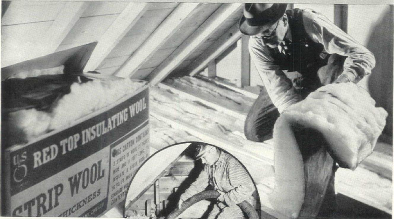
■ For the architect Red Top Insulating Wool comes very close to being the perfect insulation. It combines tremendous efficiency with low cost . . . lets the architect get the results he knows are best at a price the client can pay. A four-inch thickness has eight to ten times the efficiency of typical half-inch insulations. And the cost installed is low, so low that Red Top soon pays for itself in fuel saved.
