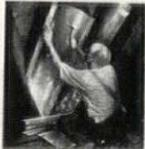
Installing Type B Metallation parallel to studs in wall.
