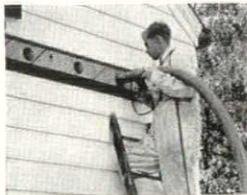
Gimco is easily blown into empty wall and ceiling spaces in homes already built.
