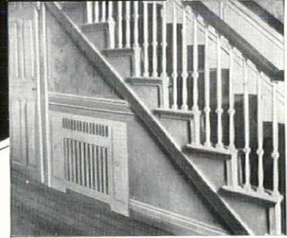
Slenderized Radiator with Radiant Front Panel.
