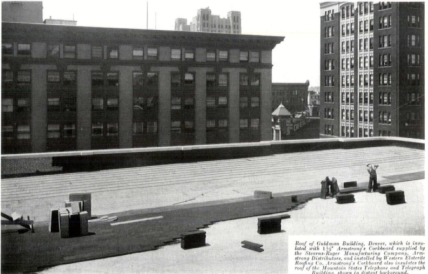
*Roof of Goldman Building, Denver, which is insulated with 1½" Armstrong's Corkboard supplied by the Stearns-Roger Manufacturing Company, Armstrong Distributors, and installed by Western Elaterite Roofing Co. Armstrong's Corkboard also insulates the roof of the Mountain States Telephone and Telegraph Building, shown in distant background.*
