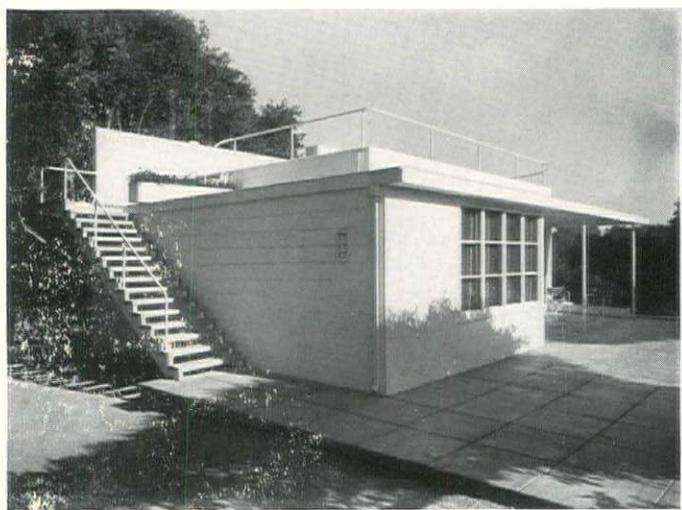
Designed as a combination guest house and recreation center, the house has accommodations for four persons. Outside stairs communicate with a sun deck which overlooks an adjoining tennis court. The construction is frame with exterior walls of flush resawn redwood siding, painted with white cement paint. The roof is a black slate mineral surfaced roofing painted with aluminum. Heating is by separate unit gas floor furnaces. All interior lighting is concealed or indirect
