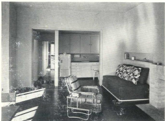
The interior walls and ceilings are of Insulite, painted a buff color. To eliminate the usual cracks and unevenness which occur when battens are not used to cover the joints, the studs and joists were spaced 2'-0" on centers to accommodate the 4'-0" widths of the material. To these were nailed 4" strips of tempered hard board, which were then coated with linoleum cement. The wall board was carefully joined with butt joints and temporarily held in place. The resulting surface was perfectly smooth
