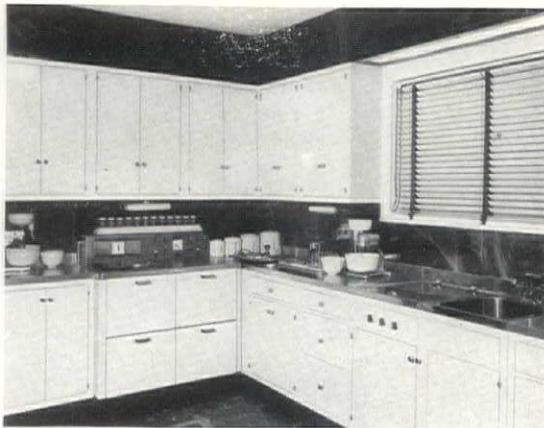
Above left: metal counter tops and range hood provide sanitary surfaces. Piping, etc., may be accommodated in furred corner. At right: note inclusion of dishwasher, lighting fixtures and convenience outlets. Sketches at extreme right show unsatisfactory door locations. Persons working at counters illustrated are endangered by swinging doors
