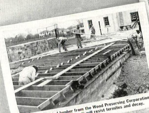
Pressure-treated lumber from the Wood Preserving Corporation (creosoted or salt-treated) will resist termites and decay.
