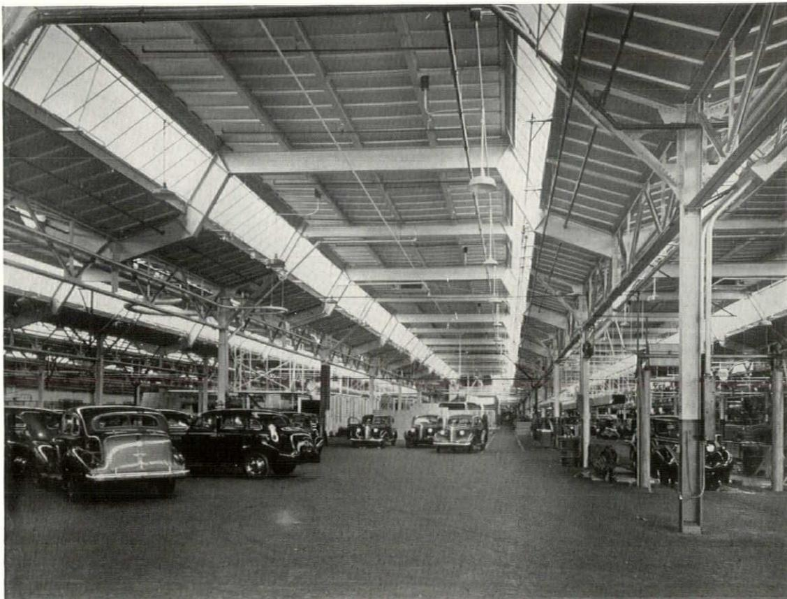
View, above, showing abundance of natural light admitted by double-monitor type roof. The well spaced columns, affording great freedom of movement, are also noteworthy. Floors throughout are of creosoted wood blocks. Below, a view of the power plant with its red and white striped smokestack rising up like a great air beacon, already a landmark in that busy industrial center.
