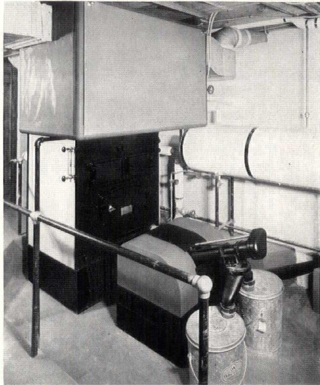
Anthracite Air Conditioning Installation. Note Automatic Anthracite Burner—feeds fuel automatically—removes ash to sealed containers.
