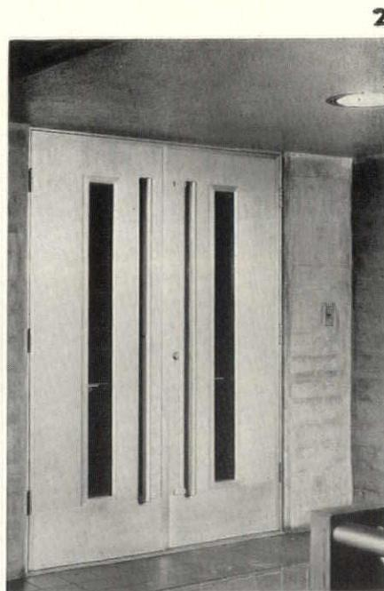
1. In rooms which house extremely sensitive instruments, this louver-paneled door is bucked up by interchangeable glass wool filters, composed of standard 6" wide units, for which the width of the louver panel was designed. The door is made in either aluminum or enameled steel.
