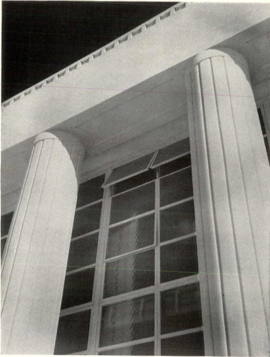
Exterior walls are of painted brick, limestone and cast stone. Partitions and insulation are of terra cotta. The interior finish is of plaster and terra cotta. Foundations are of concrete while concrete and tile are used for roofing. Floors are concrete, ceramic tile and terrazzo. Windows are steel.
