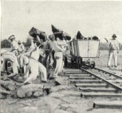
The Vital Element is dug from the surface of the asphalt lake with mattocks.
