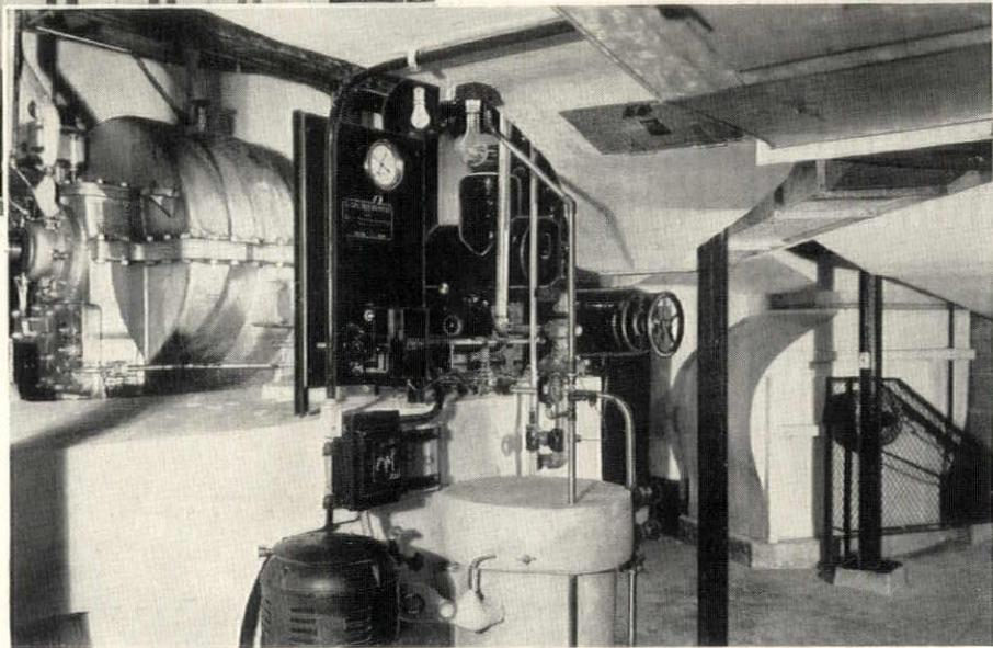
IN the modernized department store of the H. P. Wasson Company in Indianapolis, four sales floors and a basement restaurant are air conditioned. A central refrigerating system supplies cold water to several "Weather Maker" units. To prevent refrigeration losses, cold water lines in the circulating system are insulated with Armstrong's Cork Covering and Fitting Covers.
