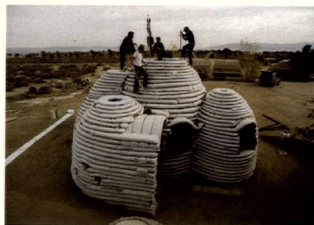
Aga Khan Award winner Nader Khalili's superadobe structures—which can be quickly built with local earth—have been used for emergency shelters in areas suffering from natural or manmade disasters.
