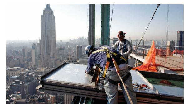
Benson's wall is a stacking system, which is designed to be erected from the bottom up, but to meet the move-in dates Tishman began installing the wall at various points up the elevation and creating what the team termed "zipper floors" where the sections meet. The unusual erection sequence allowed Equity to take advantage of prevailing market conditions and is a first for construction in New York. **AARON SEWARD**
