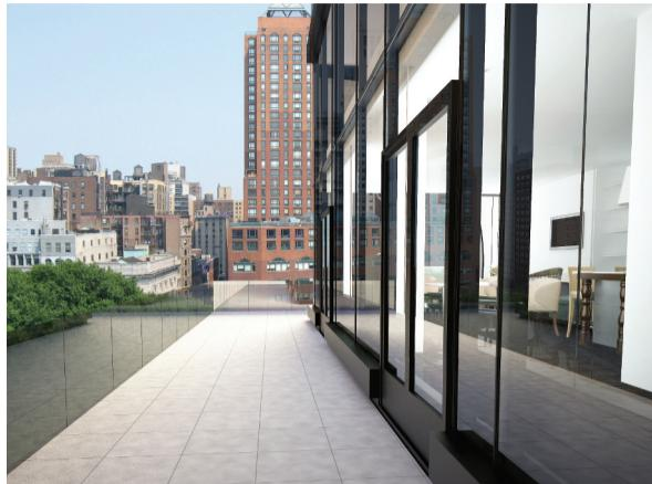
After adding seven floors to the 1870s structure (facing page, left), designers engineered a curtain wall that reveals cast-iron arches through floor-to-ceiling, argon-filled glass units (facing page, right). Setbacks create terraces with unimpeded views of Union Square, while gray-tinted, low-iron lites allow for maximum transparency (above).
