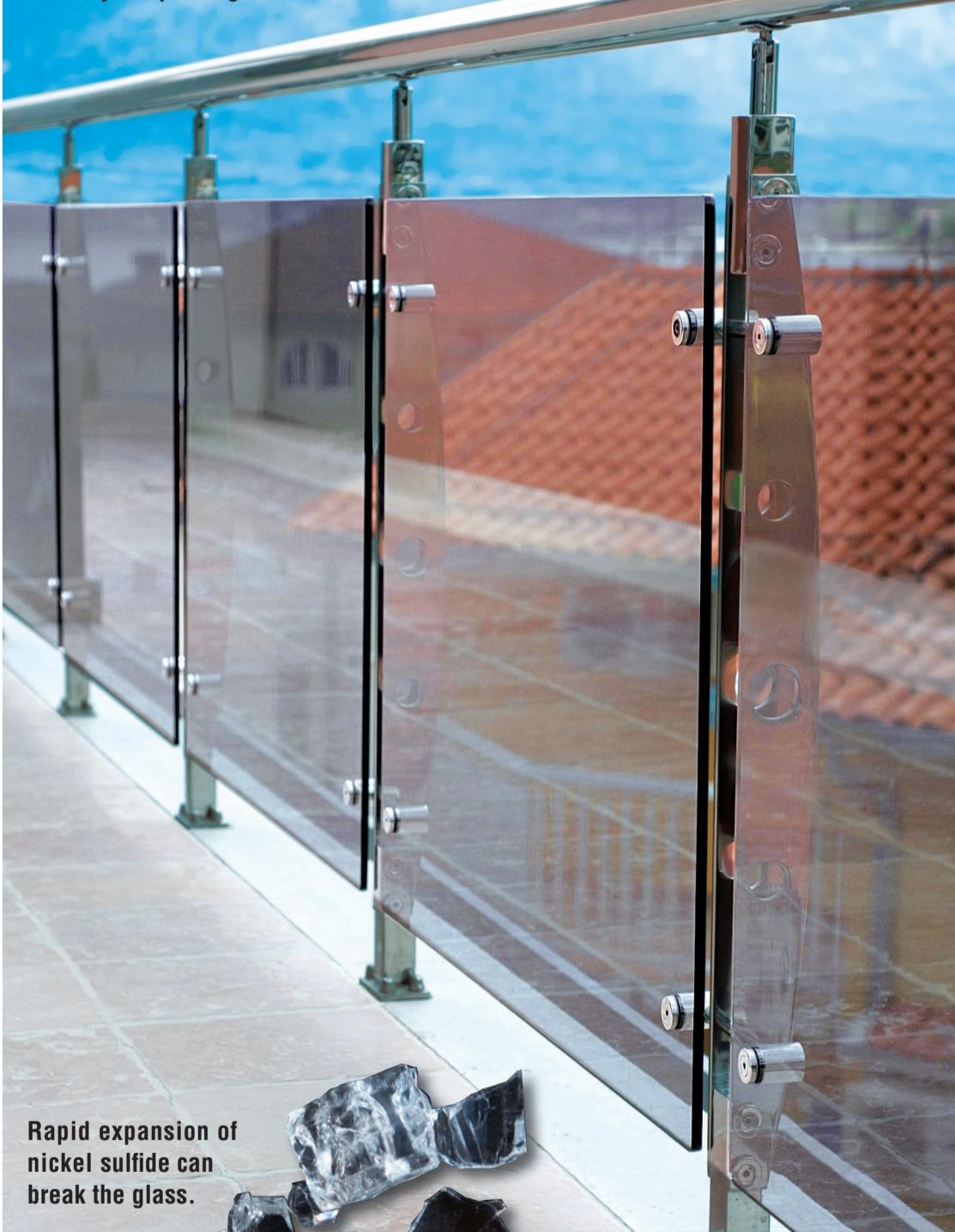
Rapid expansion of nickel sulfide can break the glass.
