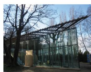
The chapel is enclosed within a lightweight glass structure (left) made of a DuPont SentryGlass Plus structural interlayer laminated with SGG Stadip safety glass from Saint-Gobain Glass. The interior of the chapel and the overall triangular shape (far left) retain the same raw but intimate sensibility of the original tent structure. The interior chapel (above) is an upturned wooden shell clad in pine strips individually steam-curved on site. DVDL
