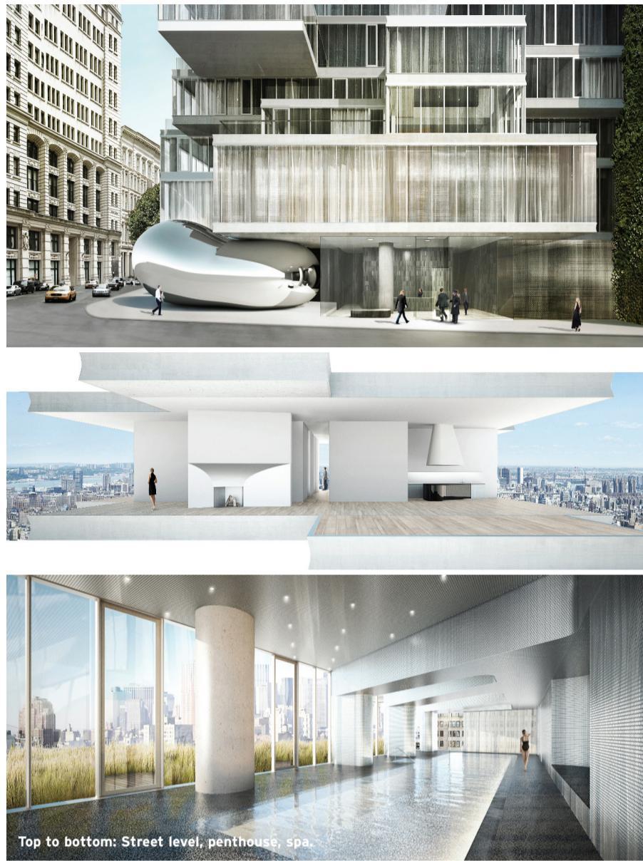
support. Most of the tower's terraces (every unit has one) hang six feet off the slab edge, though the larger ones reach out as much as 10 to 12 feet.
