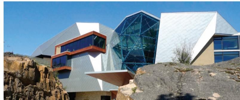
**Top and center:** The centerpiece of the Sparkling Hill Resort is a crystalline facade constructed of 15 triangles of .63-inch-thick glass, held in place by a steel armature.
