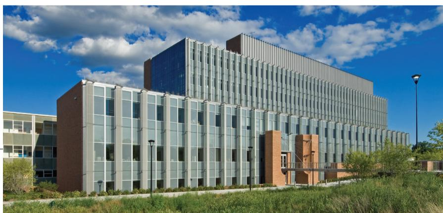
GKD-USA's metal fabric plus innovation equals ideal solar management for Eastern Michigan University: 89 stainless steel mesh panels span three varied lengths of the façade using GKD's outrigger attachment system. Solar control at every level.
