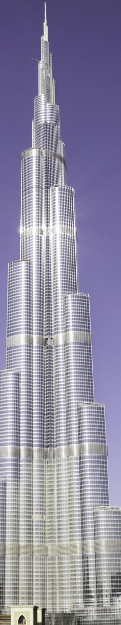
In an arid climate like Dubai's, a building's enclosure system is its most important protection against days that average a high of 108 degrees in summer. This is especially true for the world's tallest building, the Burj Khalifa, whose 2,650-foot height is clad in more than 1.8 million square feet of Guardian SunGuard Solar Silver 20 and Guardian ClimaGuard NLT Low-E glass.
