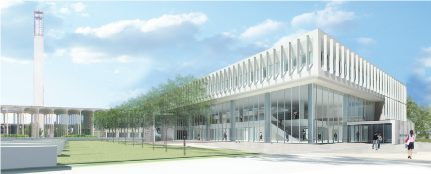
The exterior responds to Stone’s Podium with vertical precast concrete fins angled to optimize daylight. Interior “courtyards,” flooded with daylight, provide space for random encounters among students and faculty.
