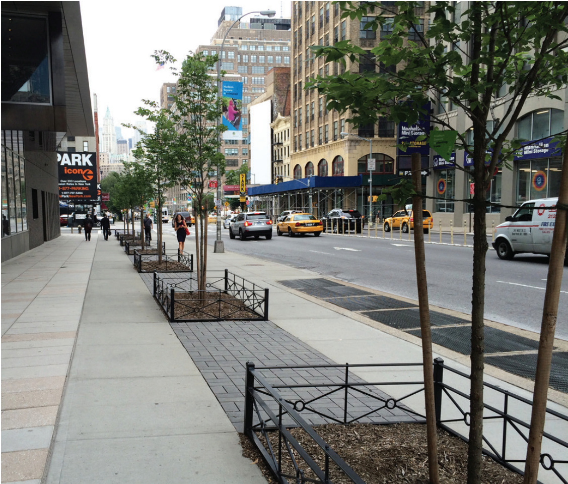
New streetscapes in Hudson Square have permeable pavers and trenches with structural soil that will capture millions of gallons of run-off; Below: The new Liberty Park Plaza, adjacent to the World Trade Center site, also designed by AECOM, will also incorporate advanced stormwater retention systems.
