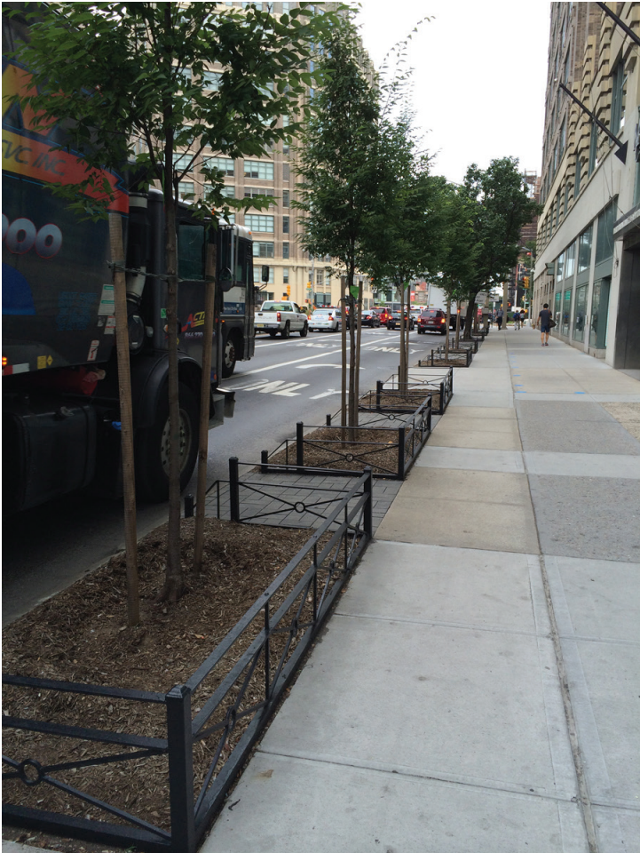
New streetscapes in Hudson Square have permeable pavers and trenches with structural soil that will capture millions of gallons of run-off; Below: The new Liberty Park Plaza, adjacent to the World Trade Center site, also designed by AECOM, will also incorporate advanced stormwater retention systems.
