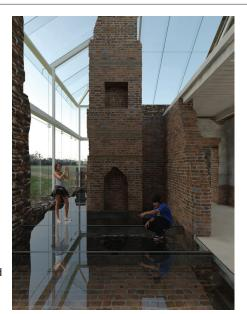
Architecture firm Machado Silvetti of Boston will preserve the decaying Menokin house with a creative laminated glass "envelope" that will protect the original structure while allowing vistors to explore the home.
