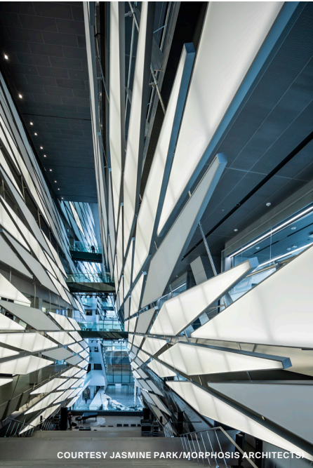
The central stairwell is lined with 400 30-foot, fiber-reinforced translucent polymer panels.
