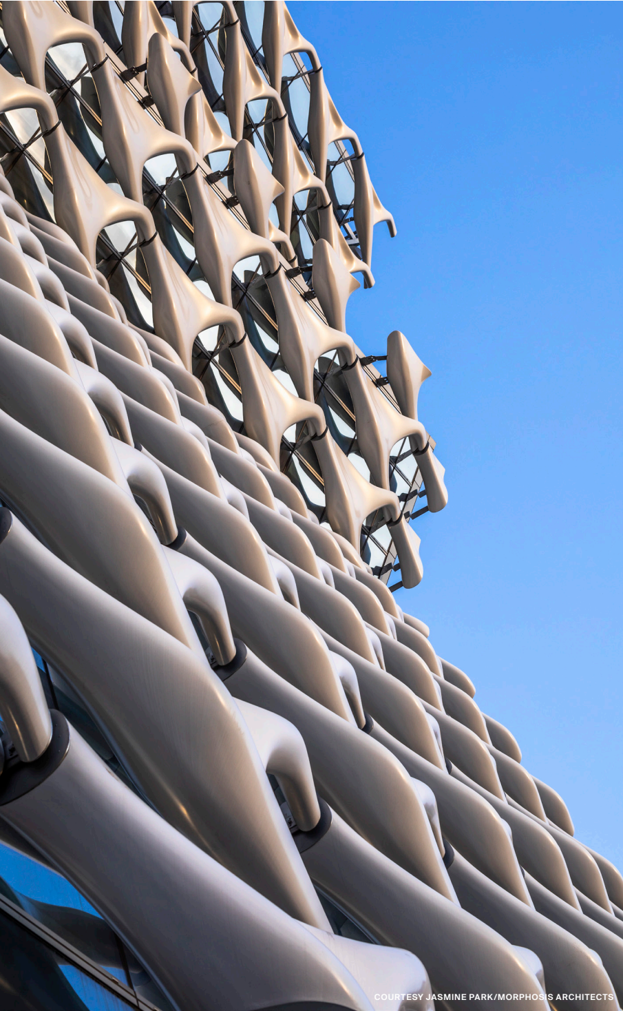
The sunscreen is composed of Aramid, a high-tech fiber manufactured by Kolon.
