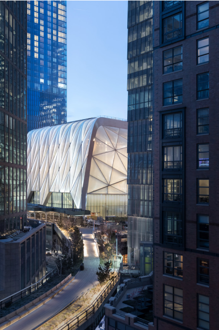
Above and above right: The doors are embedded within The Shed's movable ETFE shell. Below right: The operable doors are located on The Shed's north and east elevations. Opposite bottom: With the doors lifted, The Shed becomes an open-air pavilion. Opposite top: The guillotine doors are operated by a system of braided stainless steel wired cables that are pulled through roller bearings.
