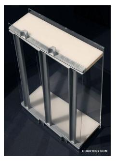
Above: Models studied the layouts of bent glass panels, left, versus flat glass panels, right. The simpler flat panels mean that the mullions must become more complex to handle the building's curves.
