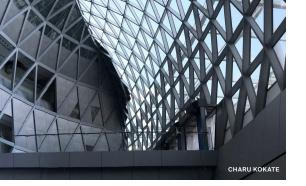
**Above:** The structural steel system is visible throughout the interior of the shopping center.
