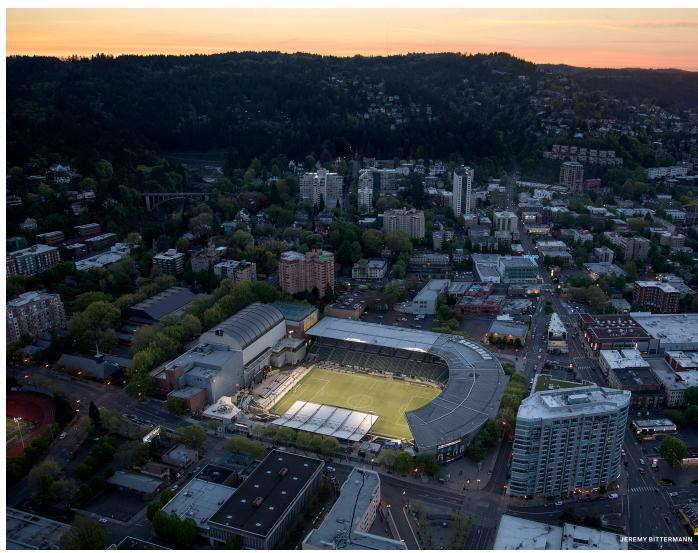
Three new levels of seating and existing stands are covered by the signature curved roof and steel trusses that wrap over the top of the structure.
