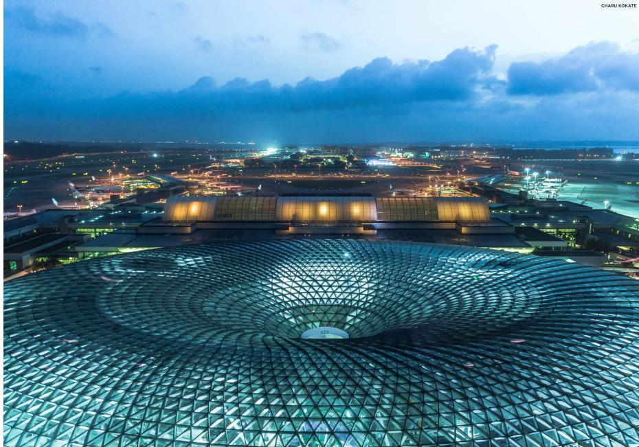
**Top:** Over 50,000 distinct parts make up the roof's stick-and-node system, which was assembled on-site.
