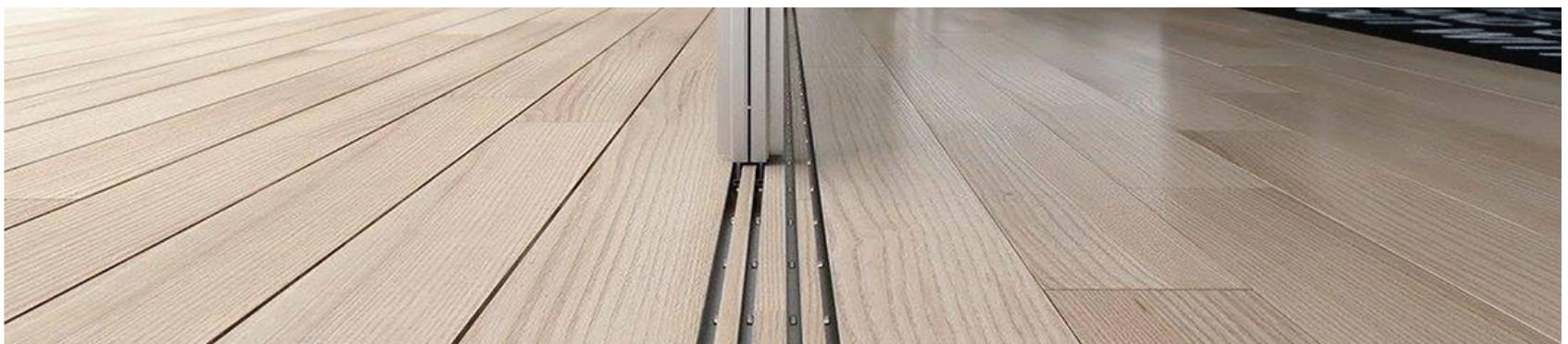
Vitrocsa's Patented Invisible Sill Option
